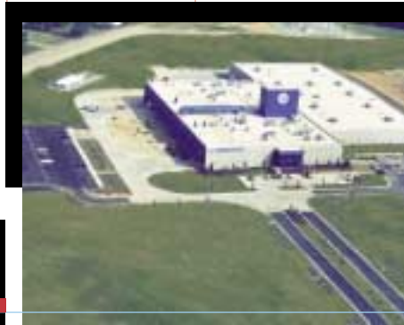
Pageland Bronze Foundry and Manufacturing Plant
